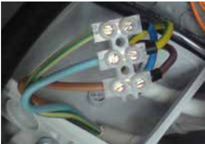
Fig. 7: Here N and PE have been reversed
