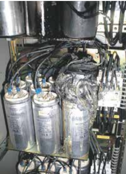
Fig.: Capacitors destroyed by harmonics current
