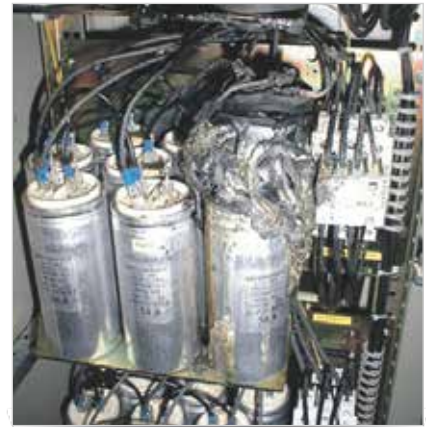
Fig. 6: Destroyed PP reactive power compensation capacitor: A creeping high-resistance short circuit to ground has caused a complete melting of the capacitor and a local fire
