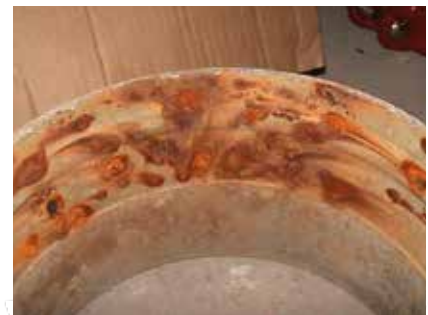
Fig.: Corrosion of pipes
