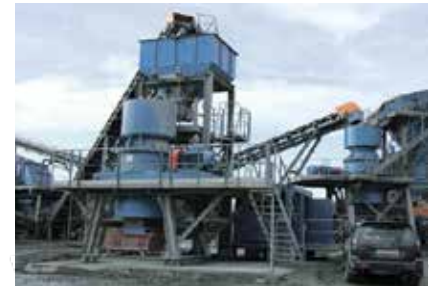
Fig.: Practical example for flicker: Gravel quarry
