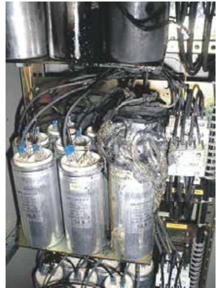
Fig.: Capacitors destroyed due to harmonics
