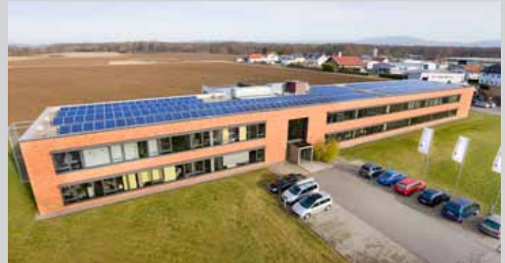
We take environmental protection very seriously: solar collectors on the roof of our building in Gottenheim generate more electricity than is required by the works.
